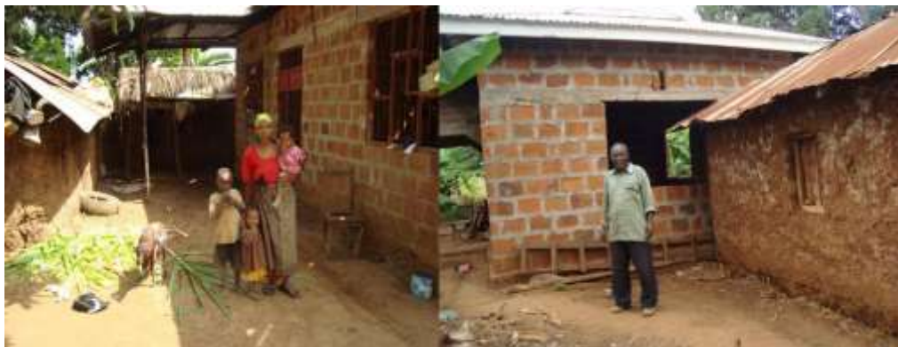
Plate 1: (Left) founding chairperson of UG depicting her modern house under construction in her left hand side and her current shelter in her right hand side. (Right) another UG member showing his modern house under construction in the background and his current shelter in his left hand side.
